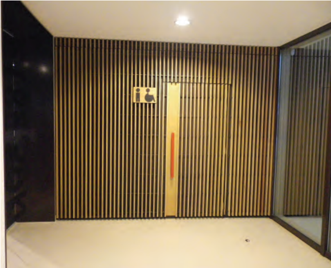
Photo: A few simple additions make this door more visible and recognizable as the entrance to the toilets in an aesthetic way. (© TGB, 2013)
