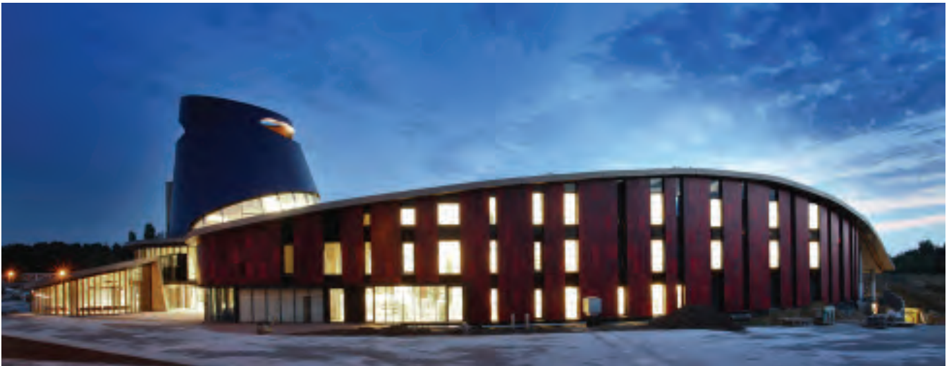
Photo: The NAC-building is not only sustainable both by means of low energy consumption, and also in its usefulness to all. (© Philippe Van Gelooven, 2013)
