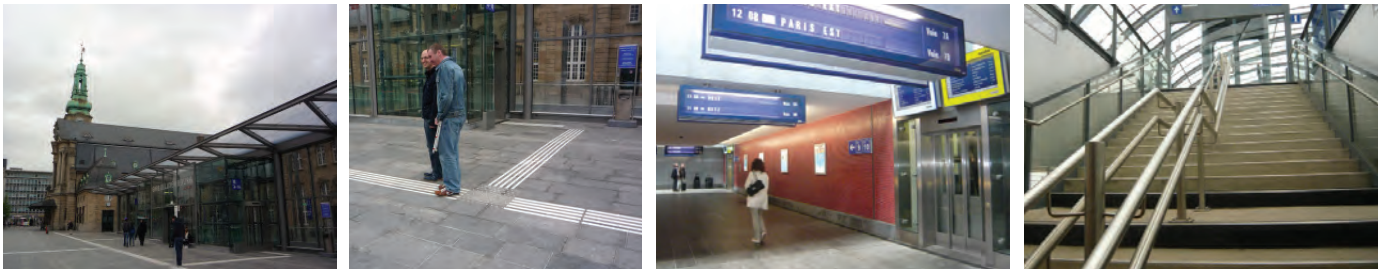
Photos: train station. Some solutions to facilitate mobility of all people: tactile signals on the pavement, lifts to reach each platform of the station, double handrails and chromatic and tactile signals on the steps. (© Isabella Tiziana Steffan, 2013)
