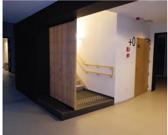
Photo: The stairs are equipped with double continuous handrails and adequate lighting. Contrasting colours and tactile markings focus attention on the steps. (© TGB, 2013)
