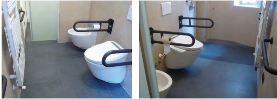
Photos: The bathroom after the works: the continuity of materials and colours, as well as the floor level in the shower area, increase the usable space, (© Isabella Tiziana Steffan, 2012)
